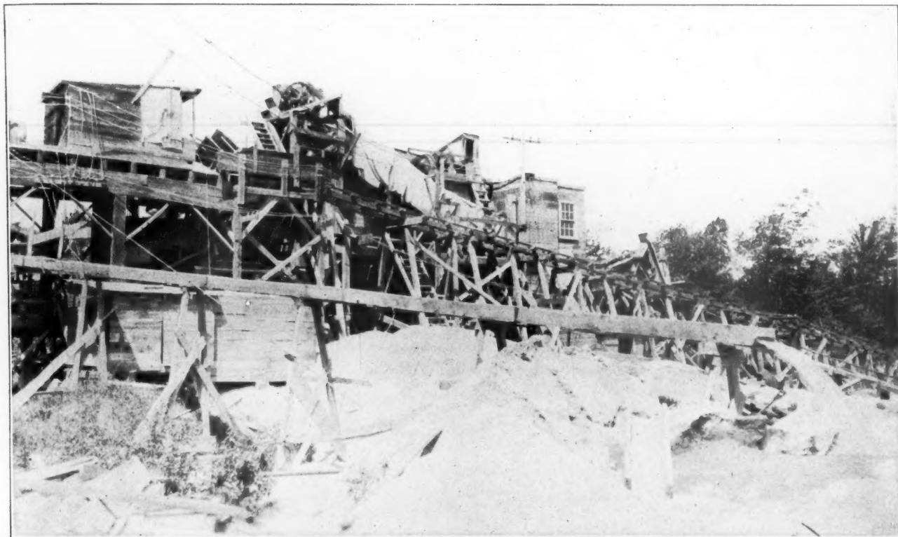
View of the Plant as a whole. Note trough in foreground which carries off water from sand settling tank.
